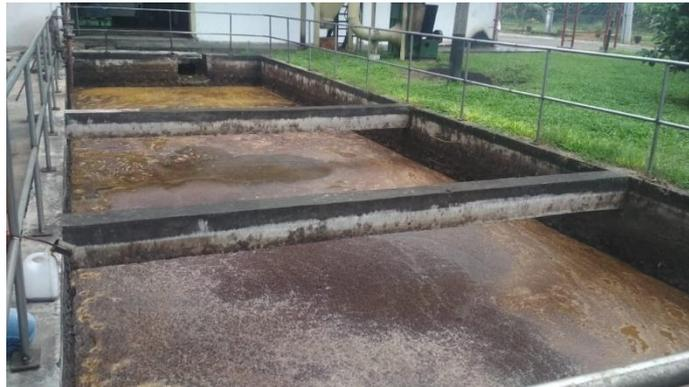
**Gambar 1. Kolam Limbah Cair Pabrik Kelapa Sawit**
